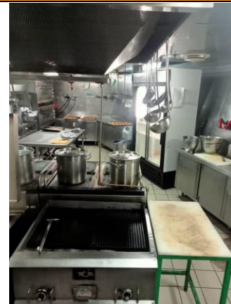
Galley – general view
