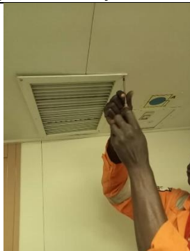
Cleaning ventilation grids
