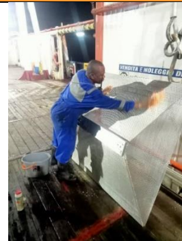
Cleaning galley ventilation hood
