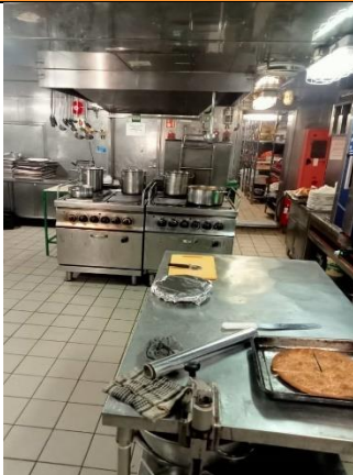
Galley – general view
